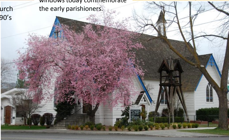
Nativty Episcopal Church 8 th Street and 8 th Ave. 2016
